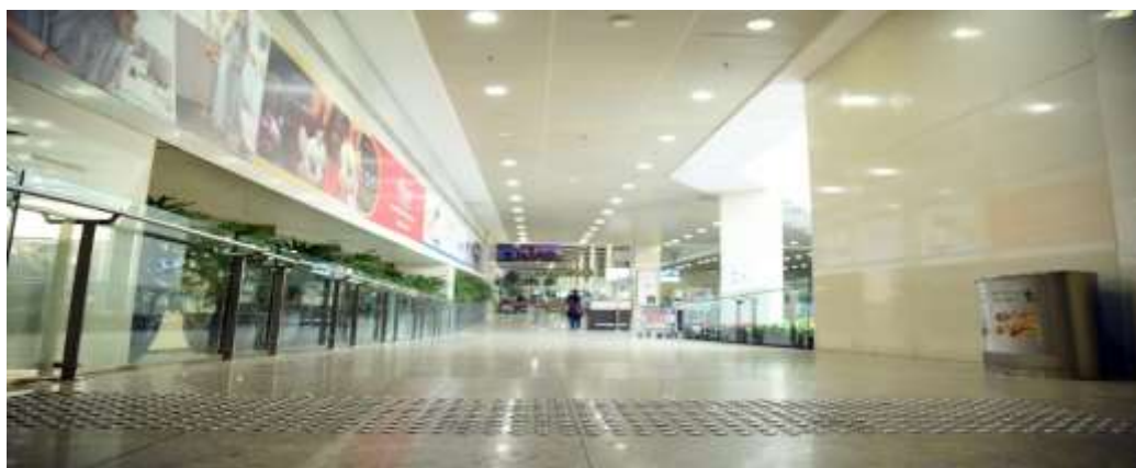
Tactile markers before and at end of ramps
